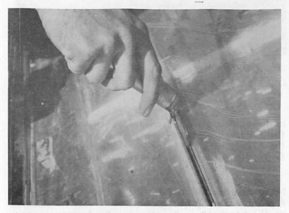
Figure 6. Polyethylene being locked into the extrusion pictured in Figure 5.
