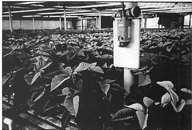
Figure 3. Thermostats and thermometers should be at plant height.
