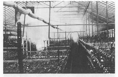
houses would normally be equipped with three 36" 1/4 HP (or 1/3 HP) fans. The owner happened to have a 48" 3/4 HP fan available. He mounted it in the center house, planning to add other fans if necessary. It wasn't.
