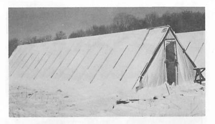
Figure 1. An early A-frame polyethylene covered overwintering structure.
