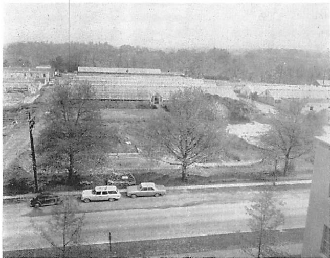
Fig. 1. Overlooking view of area of new construction. Floriculture center, Entomology left and Plant Pathology far right rear.
