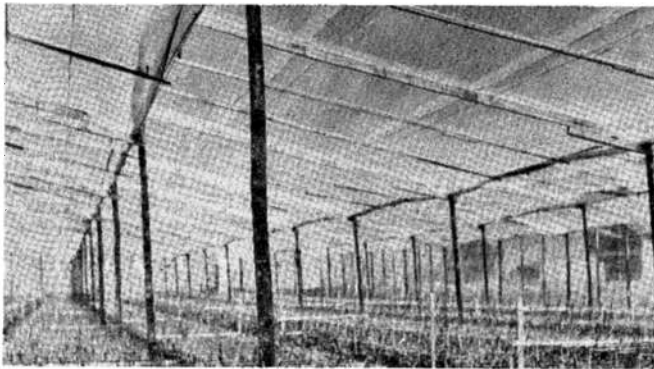
Fig. 3. Polyethylene cover for carnations as built by Clevelandia.
