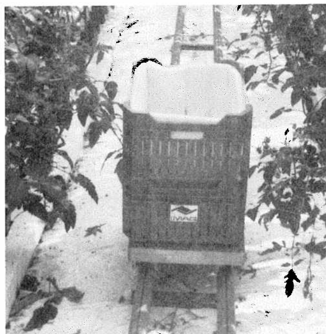
Fig. 4: Double use of hot water heating pipes. In this tomato crop, the small trolley for carrying the fruit travels over the heating pipe. No steam systems observed. In spite of more bottom heat in greenhouses, some ranges still had a lot of overhead piping — which, of course, reduces sunlight.
