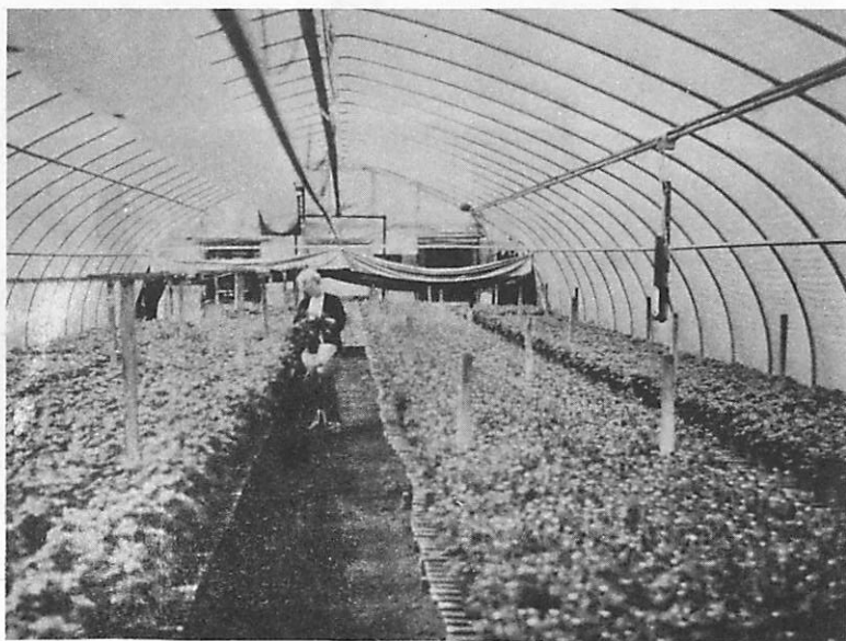
Figure 1. A double poly house with very little air infiltration.
