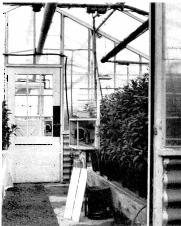
Fig. 1. Inside of one typical compartment in the CSU Temperature House, showing the centrally located, aspirated thermostat shelter with the front glass plate removed. Three thermostats separately control heating and cooling in the compartments. Temperature is monitored by two separate systems, and each compartment is fitted with its own steam condensate meter.
