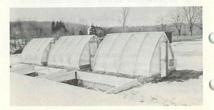
side with  $1 \frac{1}{2}$  inches of polyurethane foam insulation board. House dimensions were  $8'6'' \times 12'0''$  at the base with a center height of approximately 8 feet, giving 102 square feet of ground covered.
