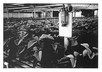
Figure 3. Thermostats and thermometers should be at plant height.
