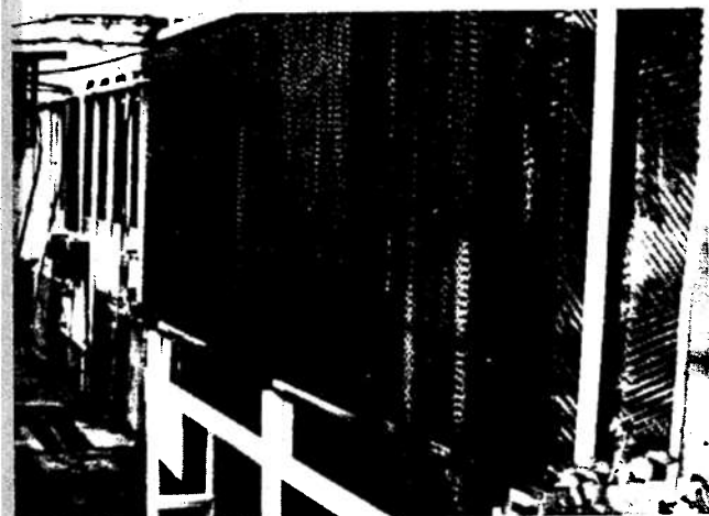
Fig. 1. CEL-DEK* pad installation using 12 x 12 x 48-inch sections.
