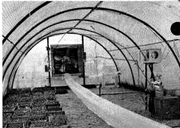
Fig. 2--Polyethylene tube in center of the quonset-shaped experimental greenhouse.
