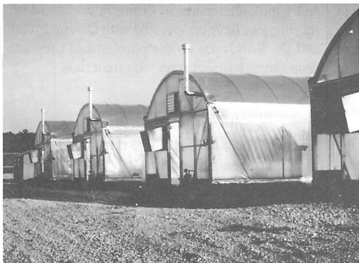
Experimental air conditioned greenhouses at NCSU. Installation of units for cooling at night to prevent heat delay in plants such as chrysanthemums may have a payback period of only 2 years.
