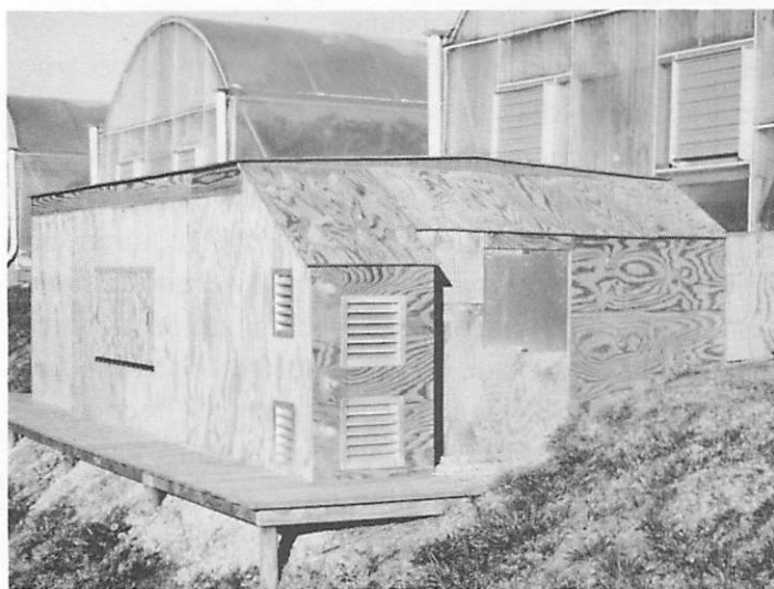
This building houses a rockbed used in NCSU greenhouse energy studies. The untapped potential of rockbeds may be their greenhouse cooling capability rather than their use in heating greenhouses.
