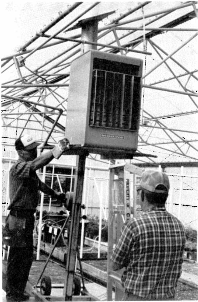
Fig. 4: Physical Plant employees removing the old, gas fired unit heaters.
