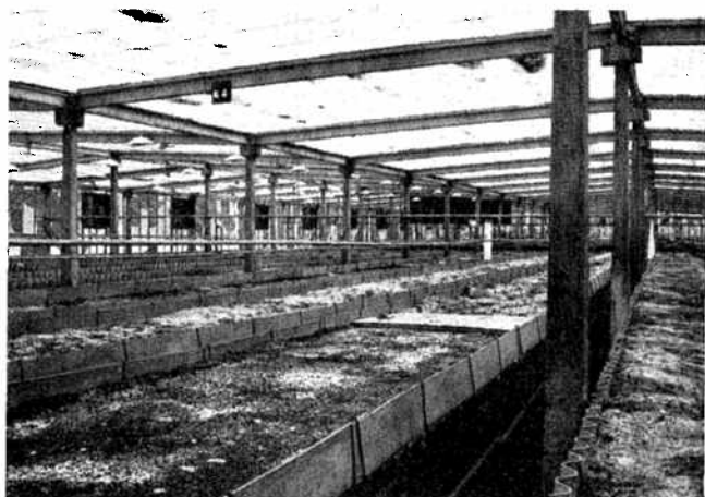
Fig. 1: Typical concrete greenhouse construction with polyethylene cover, Framptons' Nurseries, Canary Islands.
