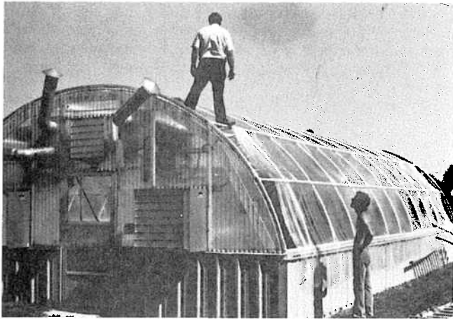
Fig. 2: Who says Professors don't work? K.L. Goldsberry on top, recovering Heat House 4 with a new Japanese, 4 mil vinyl which is as clear as glass. This will be a double film, with the heat houses planted to roses.
