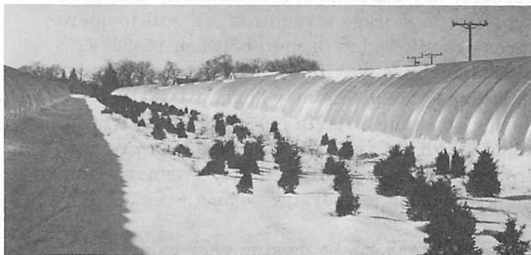
Figure 3. Large, drive-in hoop-type overwintering structures.
