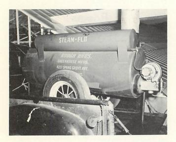
For portability, the equipment is light and easy to handle; weighing only 950 pounds empty. Mounted on pneumatic tires set to clear a 42 inch door, the boiler can easily be moved to any desired location. Consequently soil can be steamed in place, thus eliminating much time and labor ordinarily involved in soil handling.
