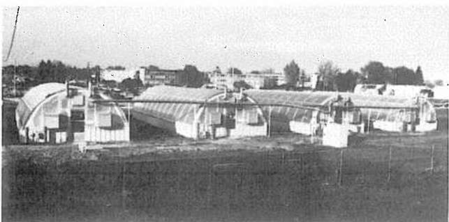
Fig. 1: CSU "Heat Houses" for climate control development. The Tectrol CO 2 duct has been removed since this picture was taken. Houses are numbered one through four from left to right, oriented north-south. Houses 1 and 3 recovered fall, 1985, so that 1 and 4, and 2 and 3 are identical.
