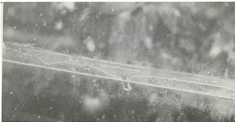
Figure 2. A "do-it-yourself" lap seal job. Very few laps were this irregular.
