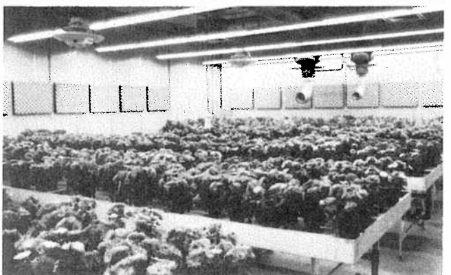
Fig. 3: Research facilities and support. Interior and outside of research greenhouses at the Plant Breeding Institute, Wageningen. All single glass, uniform installations, hot water heated, computer controlled. The total area in research glass in Holland probably exceeds the total available in these United States. The lower picture shows one of the large, post-harvest, controlled climate rooms at Aalsmeer. The waffle boards on the walls reduce the noise level.
