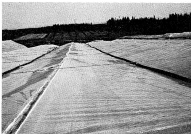
Fig. 4: Cheap plastic construction. The "ridges" are actually the walls of the house. The black tubes are filled with sand, and there are no supports under them. Support structure is minimal.
